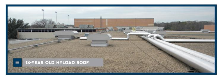
• Hyload Coal Tar Elastomeric Membranes (CTEM) were developed over 30 years ago in Europe, where they are still in use today. Hyload membranes are manufactured by a process that
